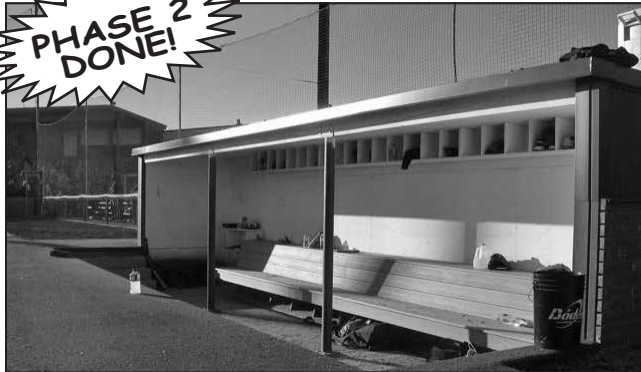
Construction of the new dugouts donated by VK Powell Construction.
